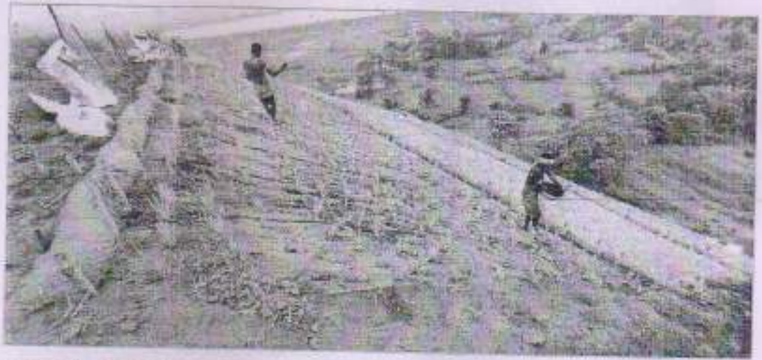
Plantation on compacted Jute geotextiles mulched area
