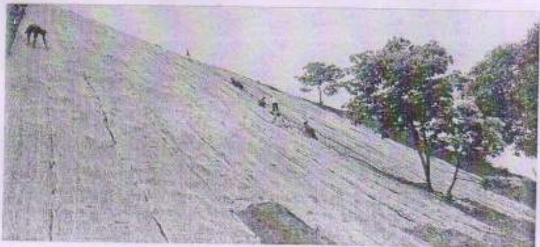
Laying of Jute Geotextiles and fixing with Bamboo pegs
